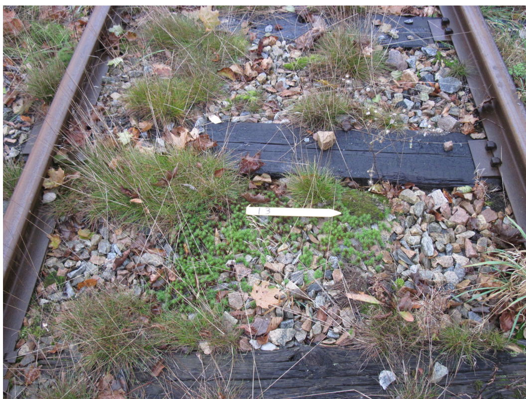
Figure 3. Weed level: ‘Increasing problem’ Biomass value 13. Weeding measures should be initiated during the season..
